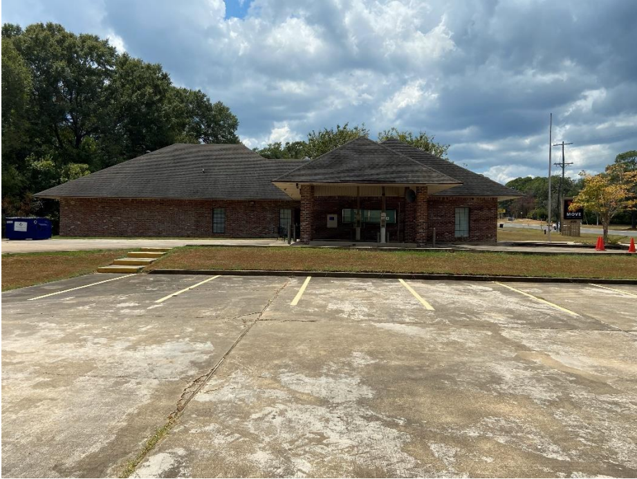
Figure 4: NE Facade of 4115 University Parkway
