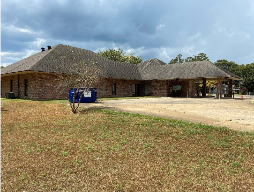
Figure 3: SE Facade of 4115 University Parkway
